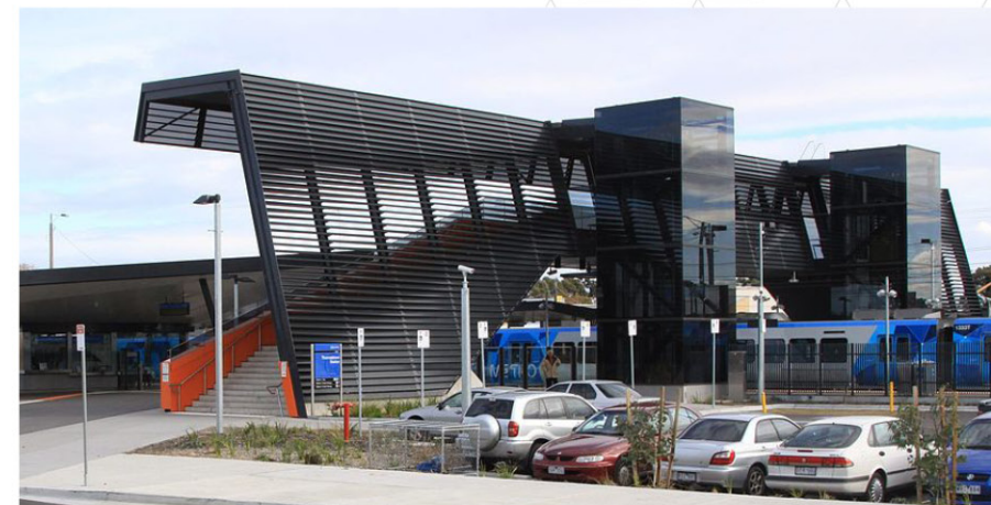
Southern Cross Station & Thomas town Station escalator, Australia
