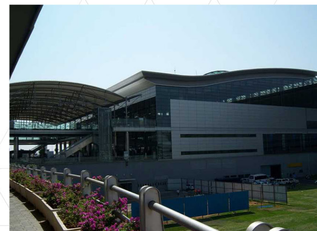
Hyderabad International Airport escalator, India
