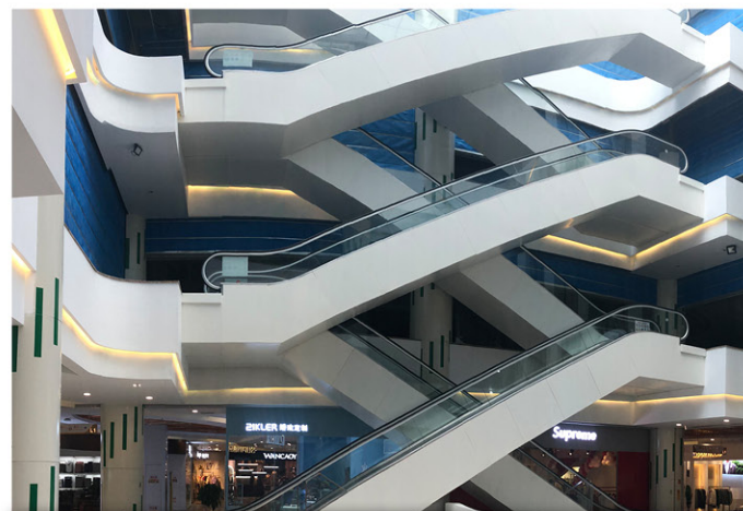
WEIHAI JIAHUA Fortune Centre Project escalator, Qingdao, China
