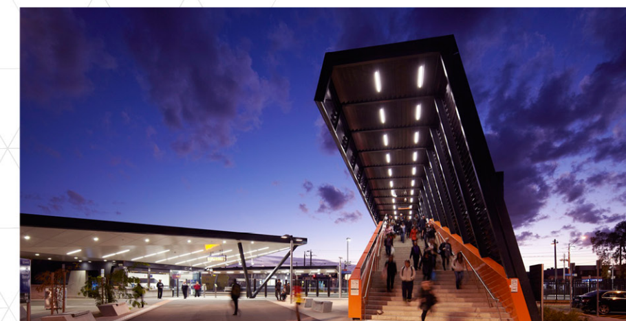
South Morang & Epping Station escalator, Australia
