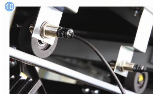
10. The escalator has electronic unintentional reversal of the direction of travel, over-speed protection device, under-speed protection device, step-loss protection device.
